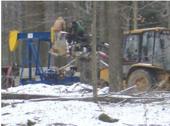
Oil workers installing a new pumpjack near the Morrison Run hiking trail in the proposed Morrison Run Wilderness Area. Photo by Jessica Ley.
